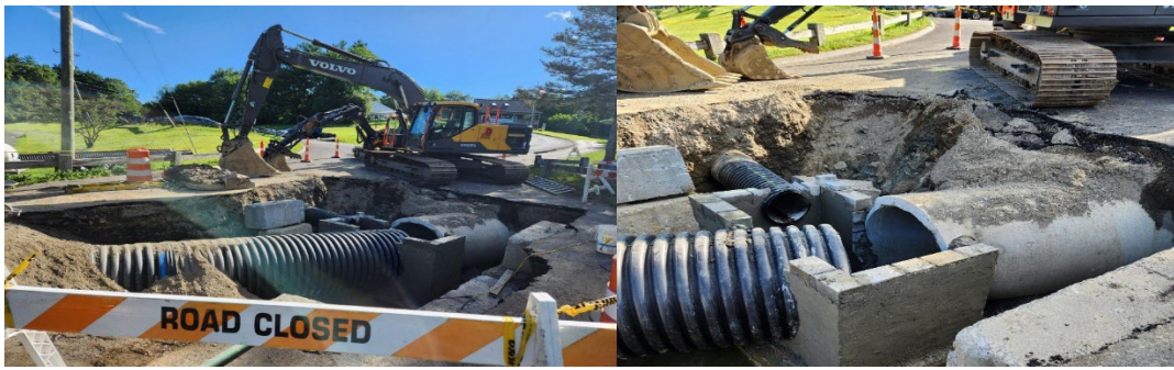
Storm Damage Repair.
